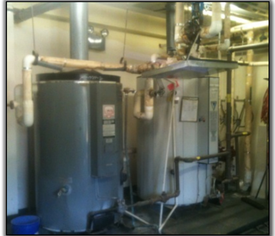
(Above) Existing 250 gallon, 500,000 Btu/hr storage type, gas-fired water heaters (Below) Existing mixing valves near ceiling with steel pan for water leaks.
