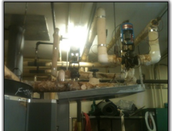
(Above) Existing 250 gallon, 500,000 Btu/hr storage type, gas-fired water heaters (Below) Existing mixing valves near ceiling with steel pan for water leaks.
